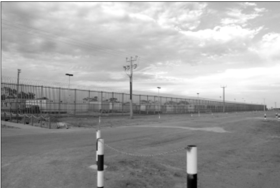
External view of Woomera Immigration Reception and Processing Centre, June 2002.
